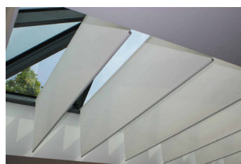
CEILING & BAFFLES RESTAURANT
