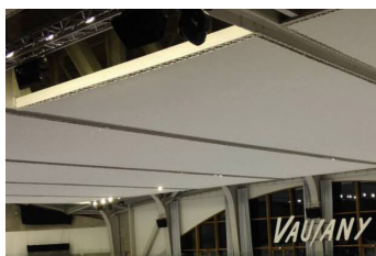
CEILING & WALLS ICE RINK
